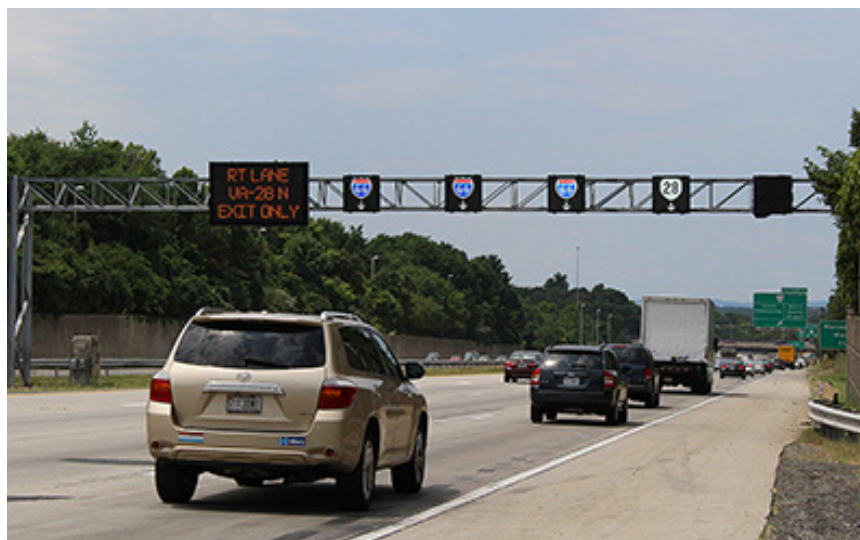
Figure 34: I-66 Active Traffic Management System Lane Control Signals in Use
